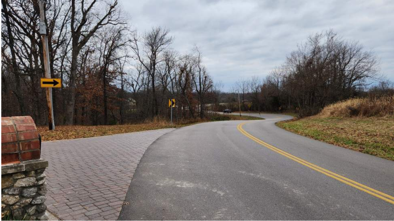
Figure 27 - Reverse curves looking to the south along Wolfrum Road.
