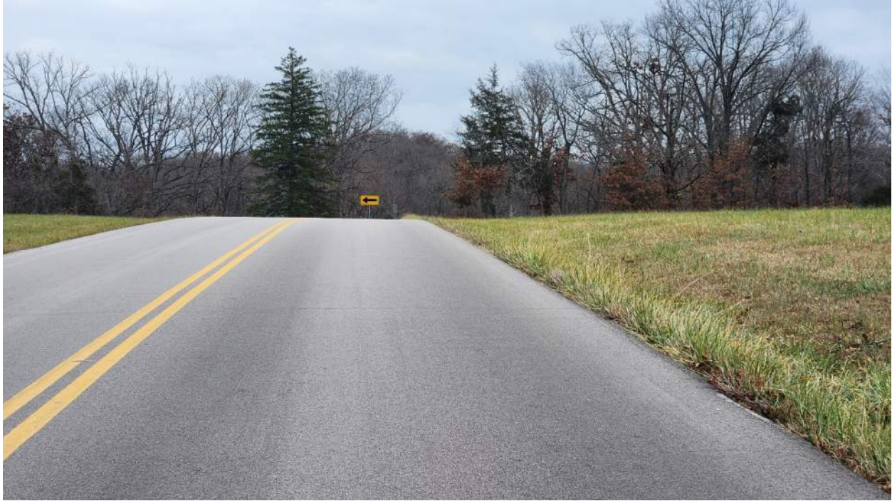
Figure 21 - View approaching the 90-degree curve at Strathalbyn Road.
