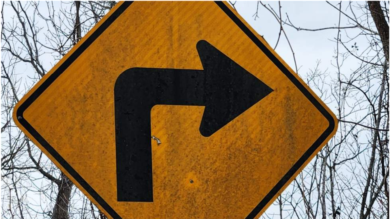
Figure 26 - Dirty sign with reduced retroreflectivity at night.
