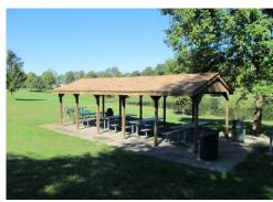
**Open Pavilion**-*Existing Conditions*: The open pavilion is approximately 30' by 15' with a wooden frame and shingle roof. The pavilion holds four picnic tables with two charcoal grills and access to electricity. The structure and picnic tables are in fair condition.
