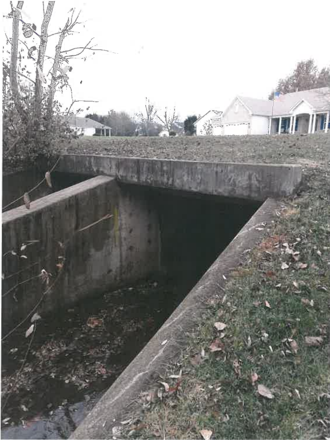
12'x8' Double Box Culvert under Wrenwyck Place Drive
