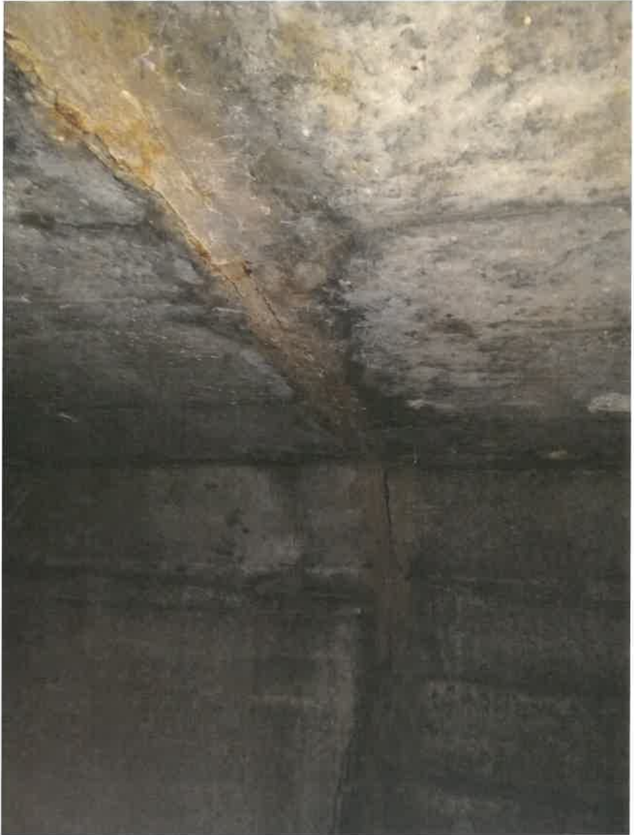
Leaking joint in Box Culvert
