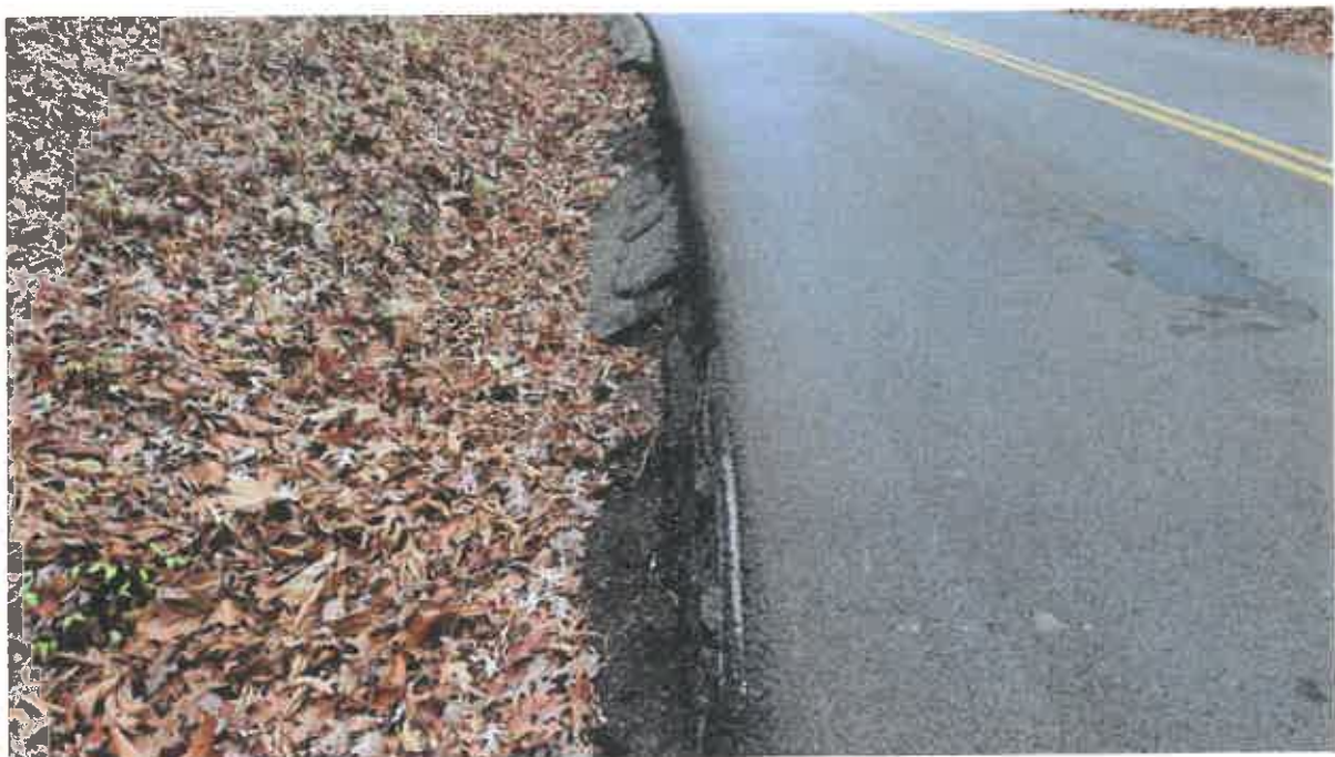
Figure 29 - Pavement edge drop-off east of Patriotic Trail
