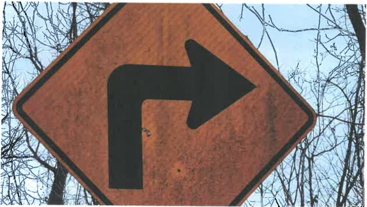
Figure 26 - Dirty sign with reduced retroreflectivity at night.
