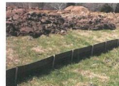
Silt Fence or Straw Bales shall be properly staked around the lower side of any open excavation to prohibit sediment from leaving site.
